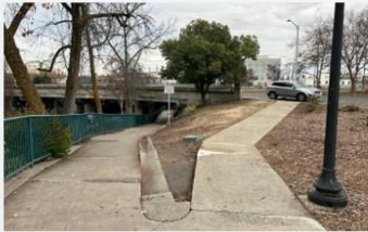
Sidewalks along Washington Boulevard.
