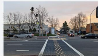
MEDIAN REFUGE ISLAND
