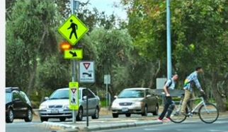
RECTANGULAR RAPID FLASHING BEACON
